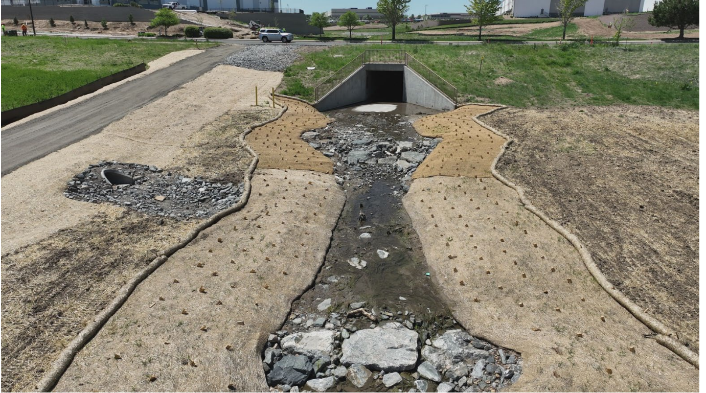
Figure 6: Downstream of Chambers Road (Looking Upstream) – Courtesy of SEMSWA
