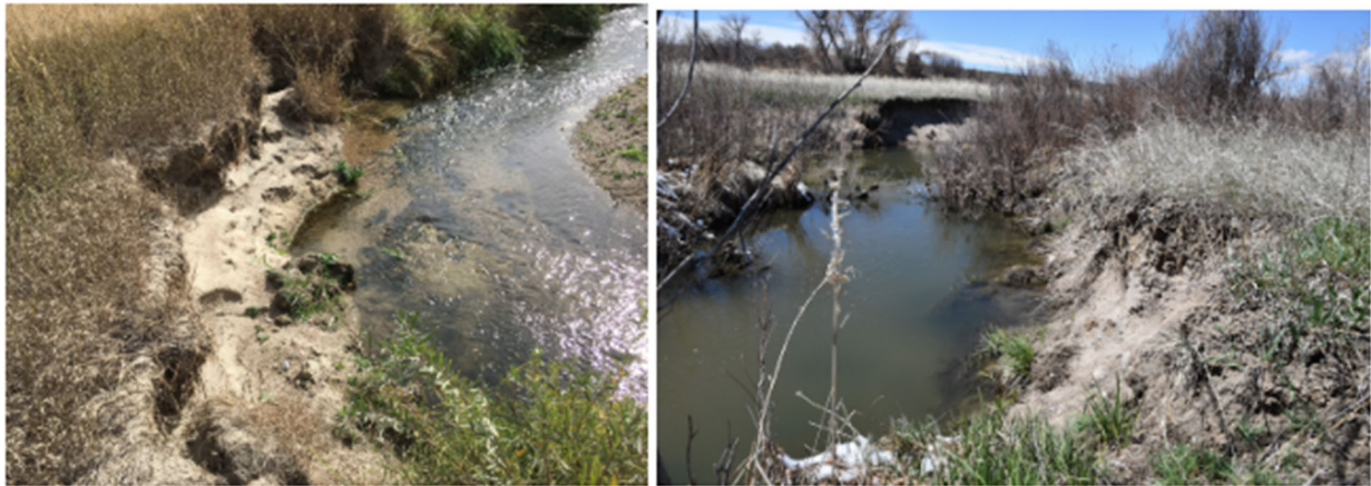
Figure 13. Before photo of the Cherry Creek at Scott Avenue project
